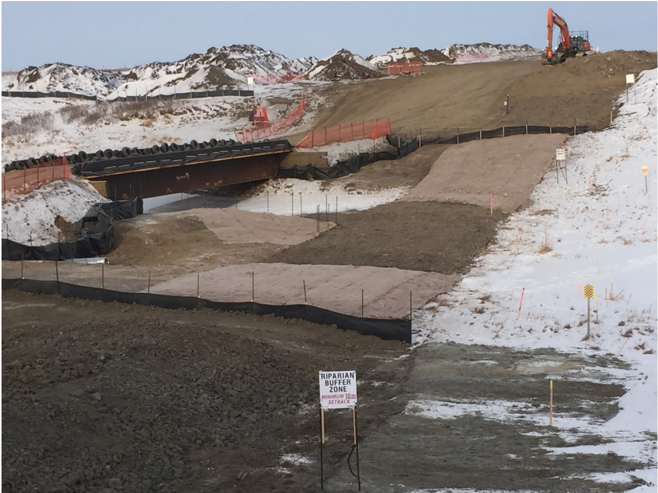
HIGH HILL AFTER RESTORATION.
