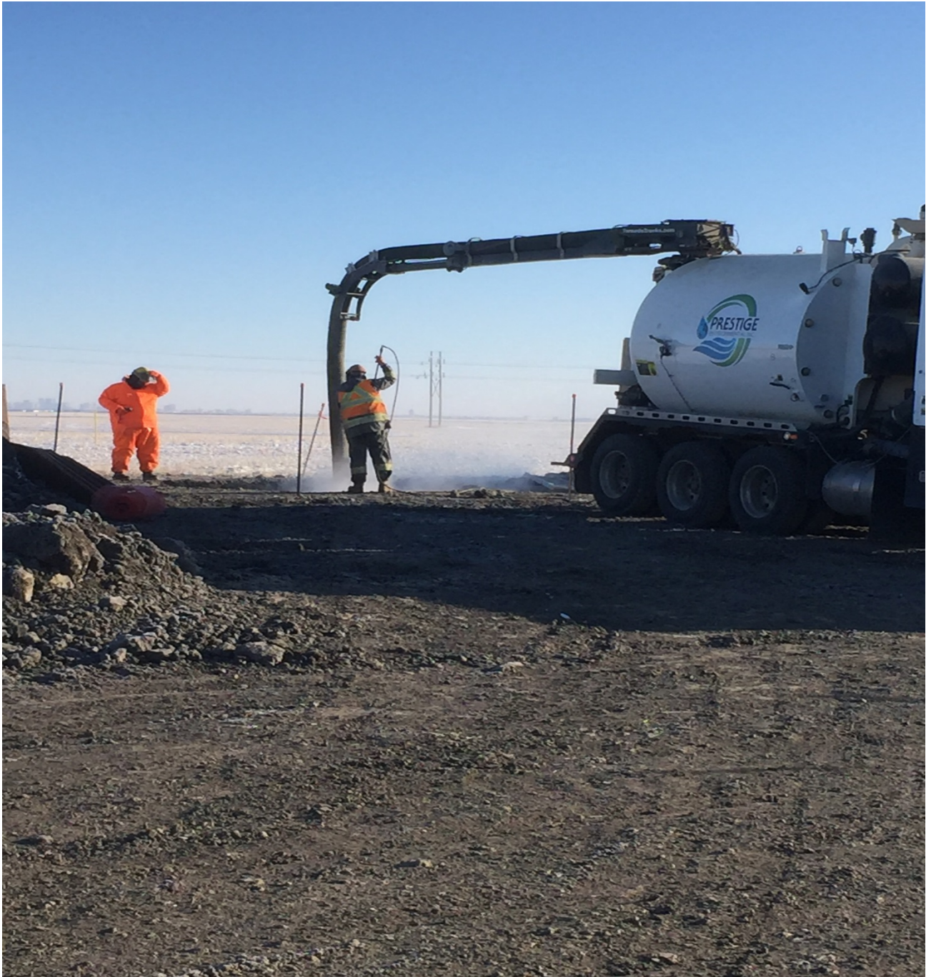
HYDROVACS LOCATING EXISTING LINES AT TRANS CANADA HIGHWAY.
