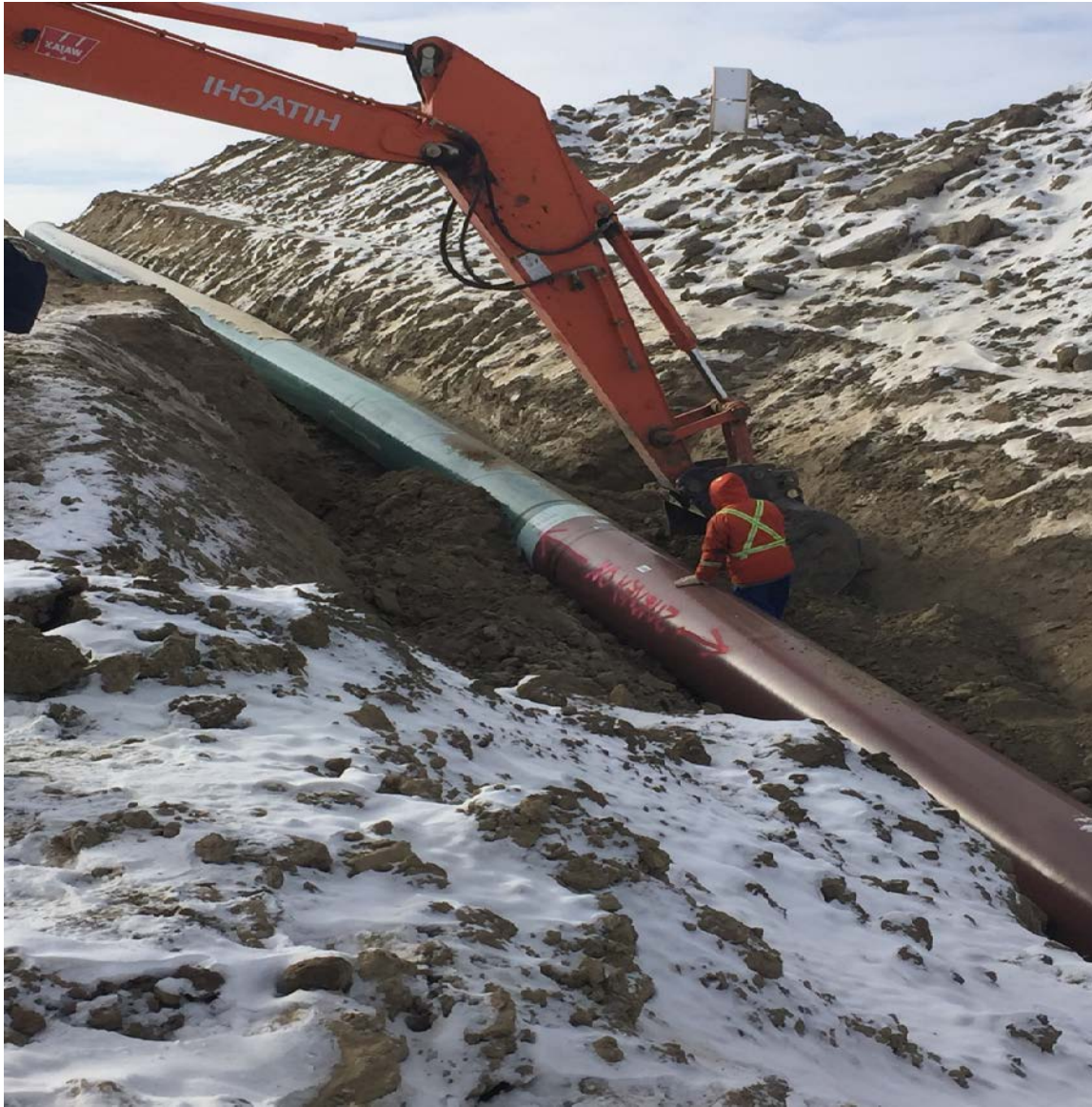
BACKFILLING PIPE WHILE IT IS IN THE TRENCH.
