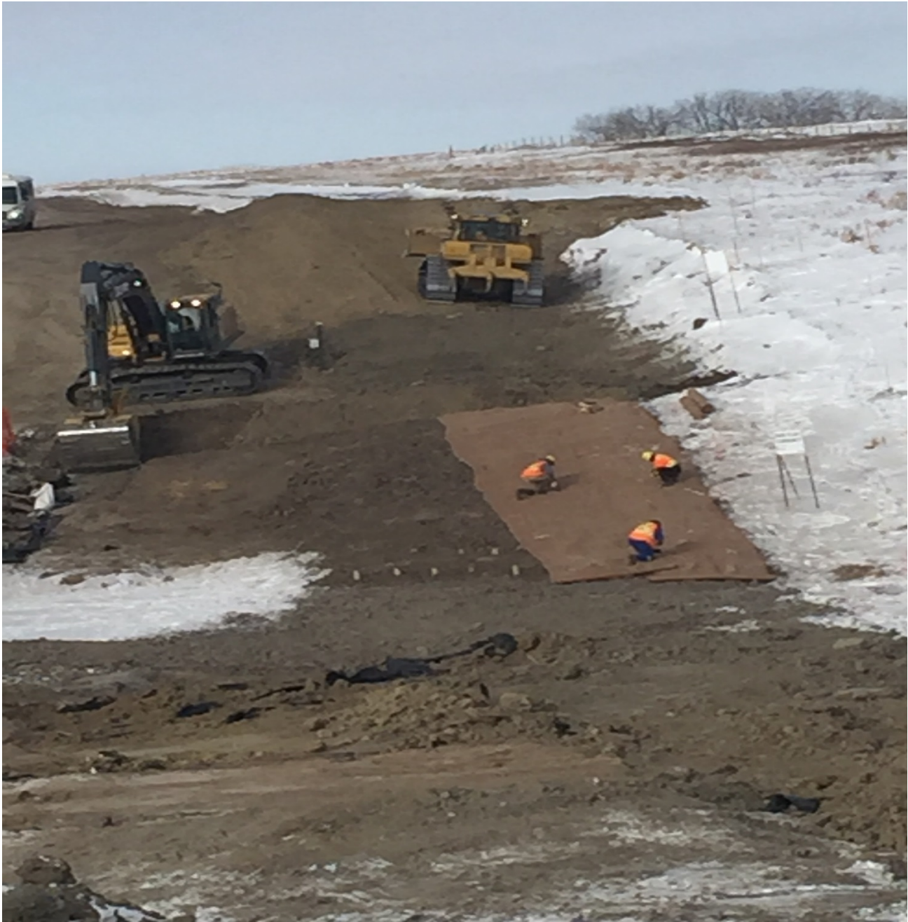
WORKING ON CREEK RESTORATION.
