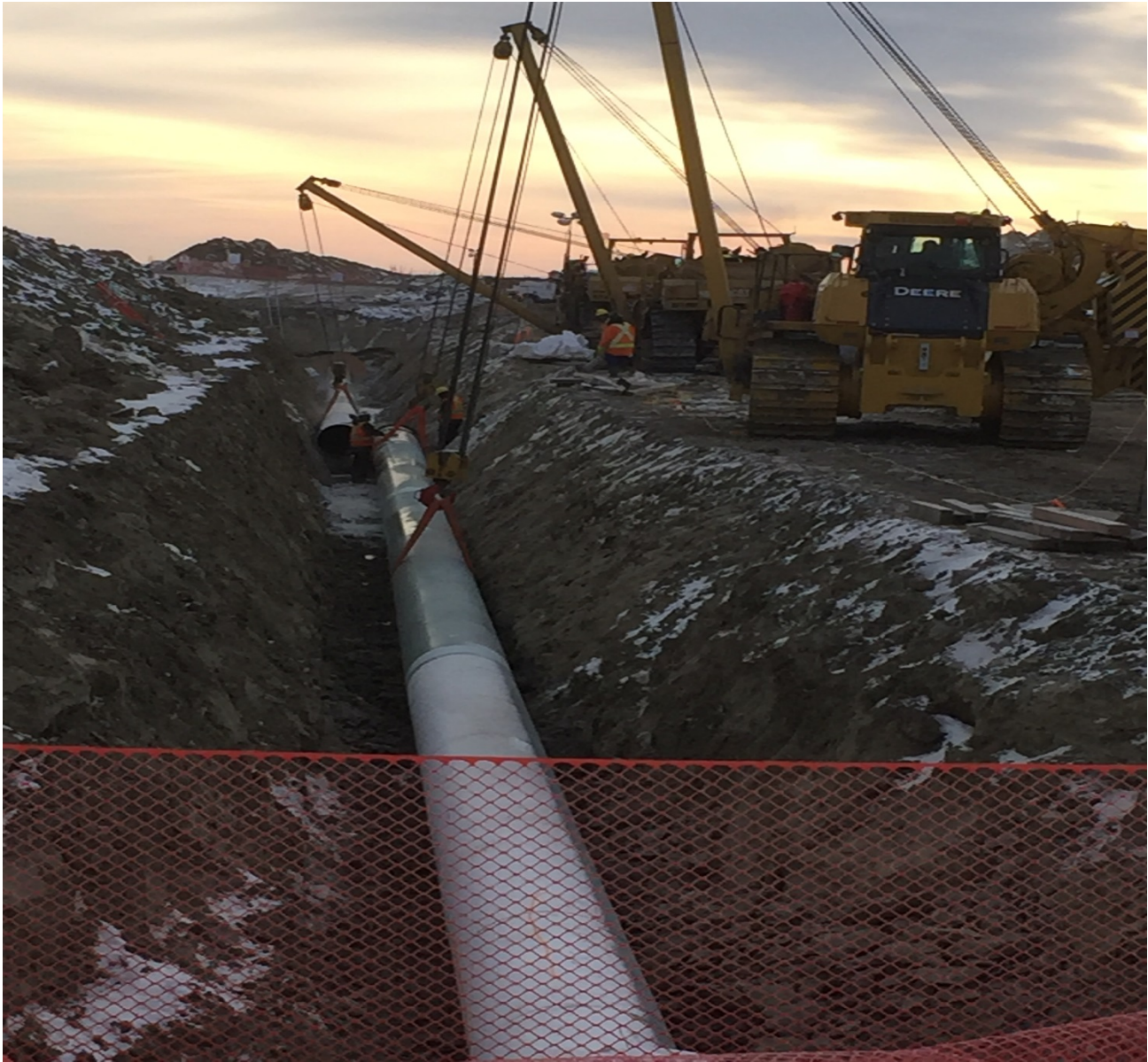
EARLY MORNING PIPE LOWERING.
