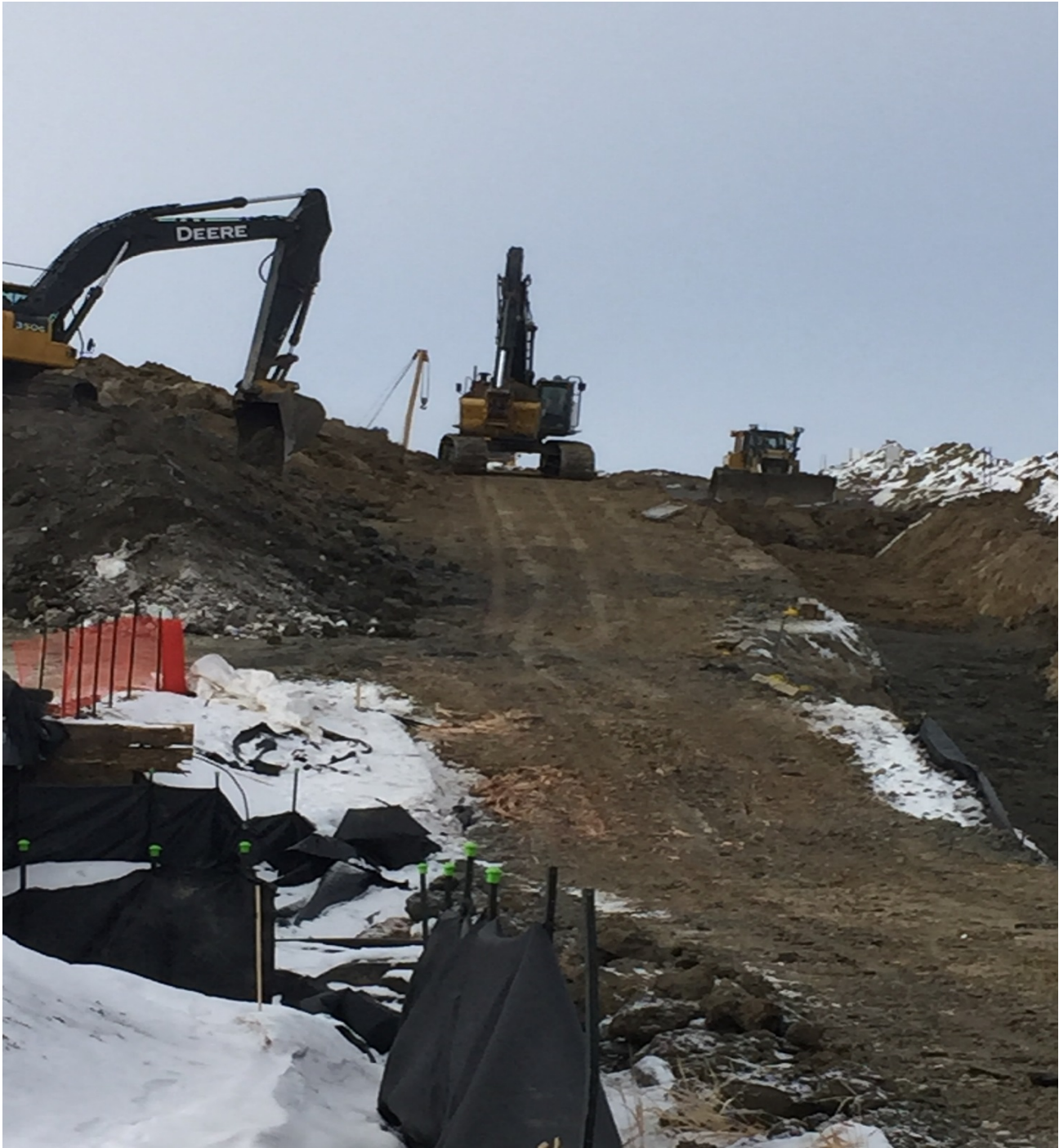
COTTONWOOD CREEK GETTING BACKFILLED.
