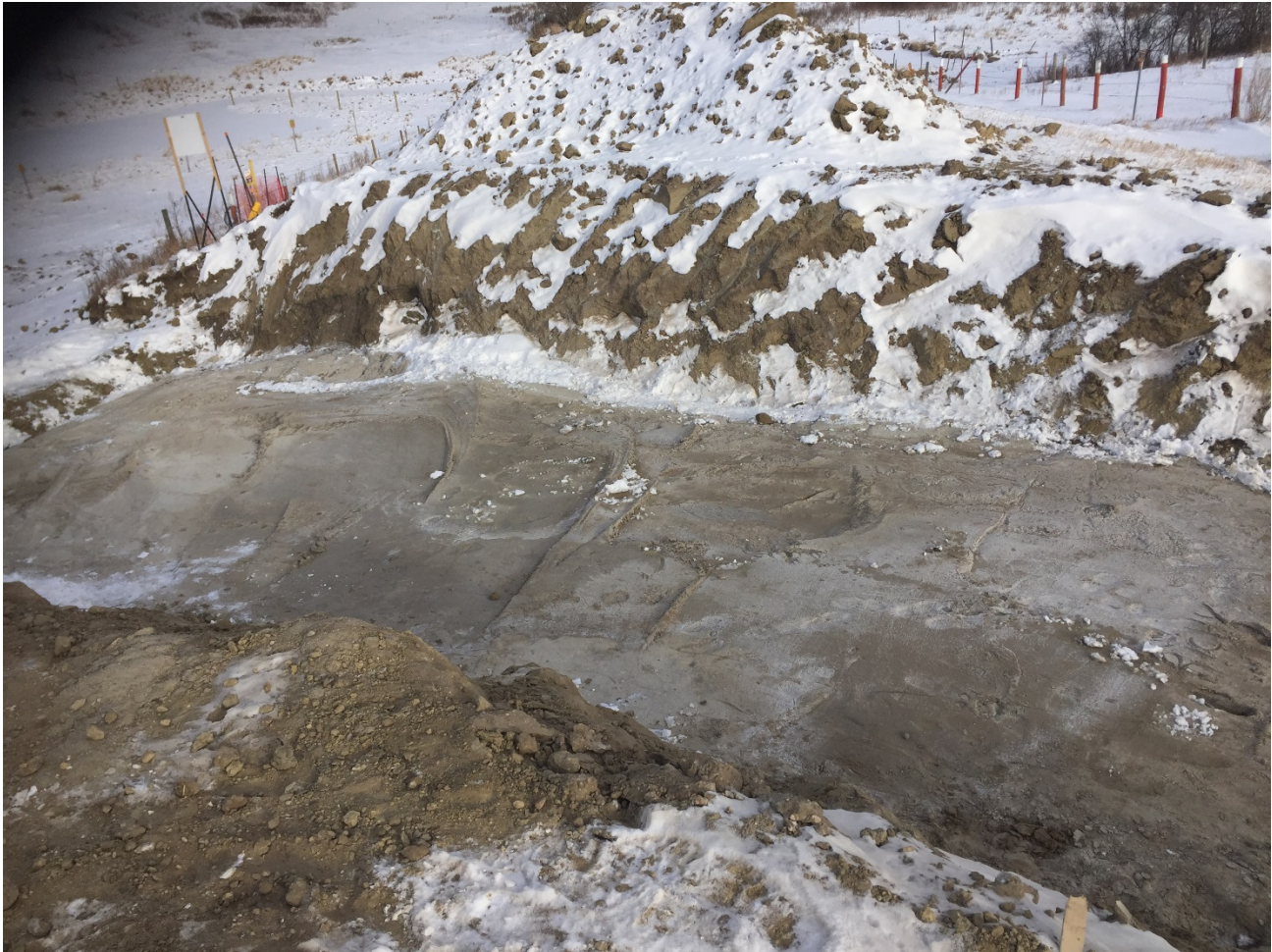
FILLCRETE THAT HAS SET ACROSS OPEN CUT ROAD AT HIGH HILL CREEK.
